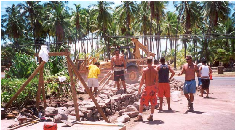
Billy Fields (on right) teaching dry-stacked rock wall construction at Kulana O'iwi , Moloka'i
