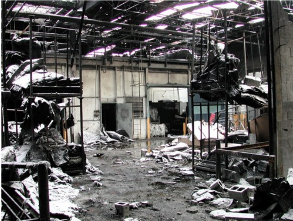
Figure I-2: Results of a dust explosion at CTA Acoustics, Inc., on February 20, 2003. (Source: CSB)
