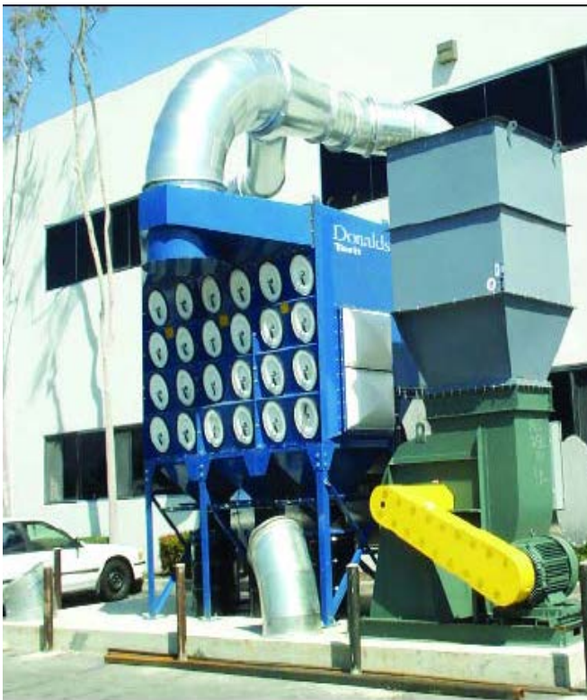
Cartridge and Envelop Baghouse (Source: Donaldson Co.)
