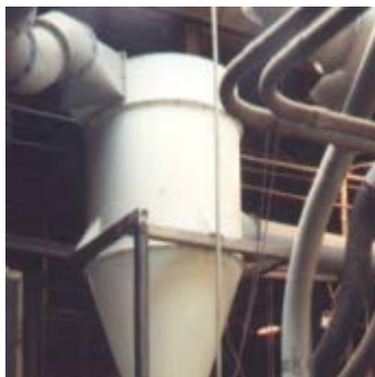
Cyclone Dust Collector (Source: OTI)
