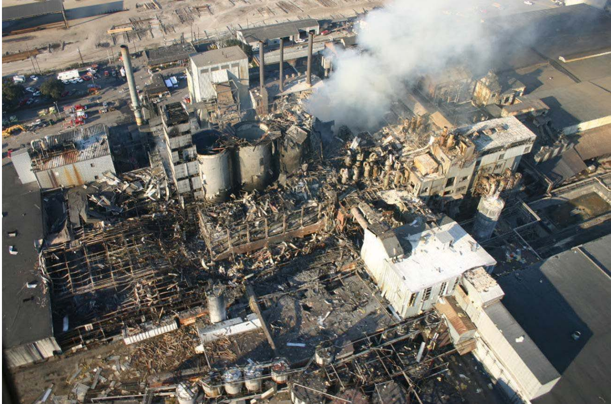
Figure I-4: Results of explosions and fires at Imperial Sugar Company on February 7, 2008. (Source: CSB)
