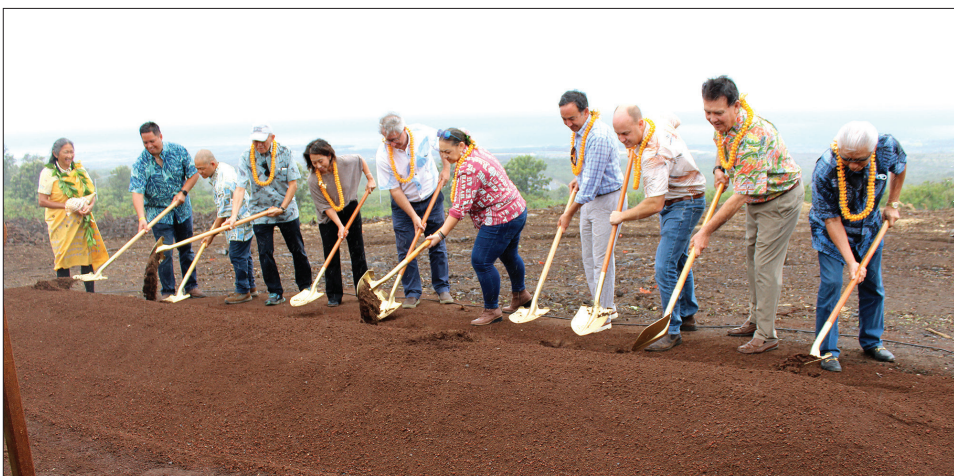
Officials and dignitaries break ground Friday on the Kaloko Heights Affordable Housing Project. LAURA RUMINSKI/WEST HAWAII TODAY
