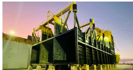
Commercial - Alt. Energy
